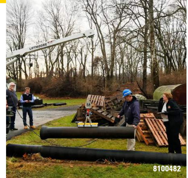
Lifting Pipe with MLAY1000x6 Lifting Magnet
