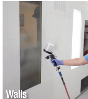
Walls Apply 3M™ Booth Coating on walls.
