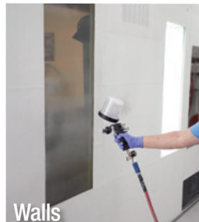
Walls Apply 3M™ Booth Coating on walls.
