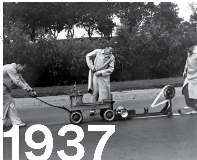
Engineer Harry Heltzer, started “The Glass Beads Project” to develop a centreline material that was more visible than paint.
