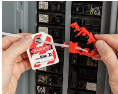
Save time by "pre-loading" your tag and cable tie before walking to the energy point
