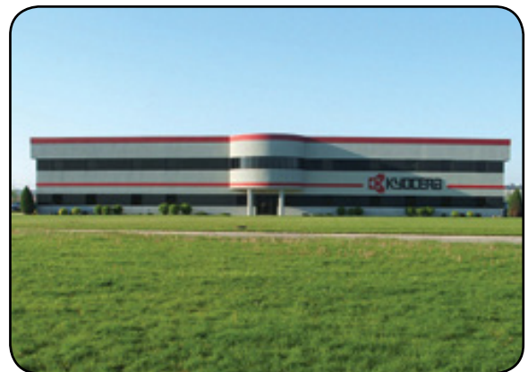
KICC, Cutting Tool Division Ohio Production Facility Wapakoneta, OH
