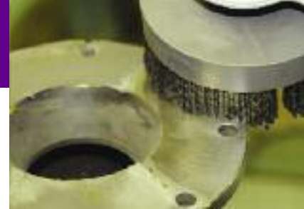
Removing gasket material from a pipe flange.
