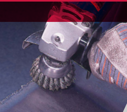
Removing slag from a flame-cut Steel plate.
