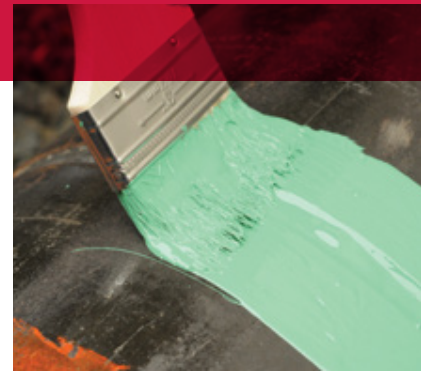
Applying pipe coating to weld seams.
