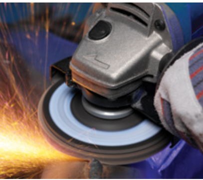
Blending and finishing a weld.
