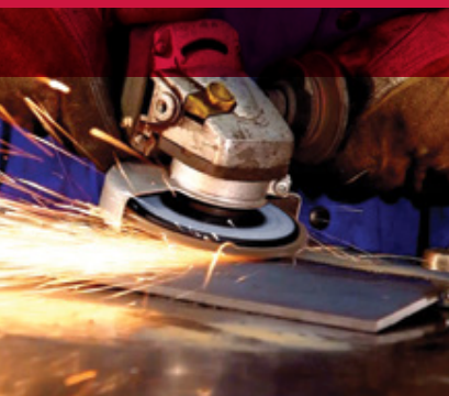
Grinding & blending a weld between two Steel plates.
