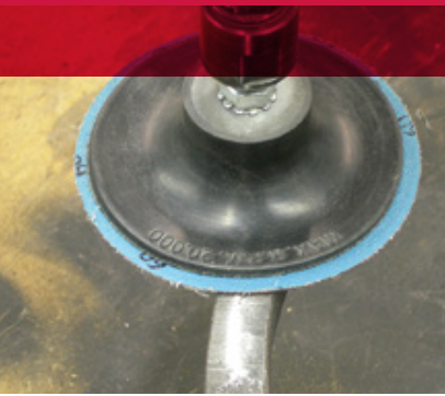
Blending surface imperfections prior to painting.
