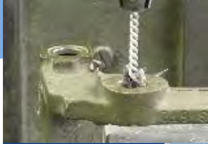
Removing zinc coating from holes in a brake bracket.
