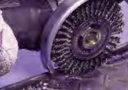
Cleaning a weld with a stringer bead wheel brush.
