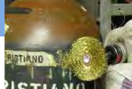
Removing labels from a compressed-gas storage cylinder.
