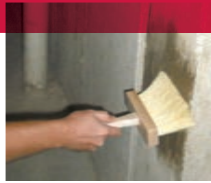
Applying waterproofing material with a masonry brush.
