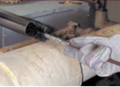
Cleaning boiler pipes with a flue brush.
