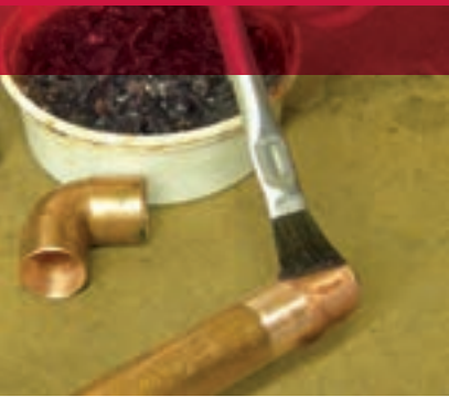
Applying flux to a copper tube prior to soldering.
