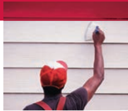
Applying paint to clap board siding.
