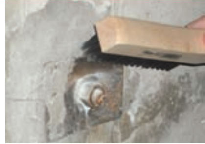
Removing excess concrete from the surface of a steel support plate.
