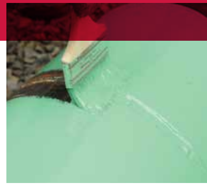
Applying pipe coating to weld seams.
