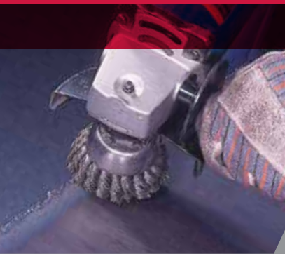
Removing slag from a flame-cut steel plate.
