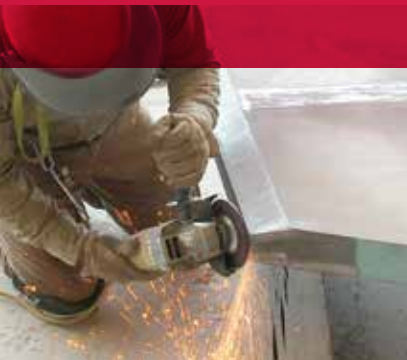
Grinding on a platform for weld preparation.
