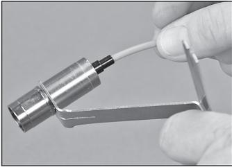
8.19 Slide the metal crimp ring onto the back of the connector, capturing the Kevlar.® fibers
