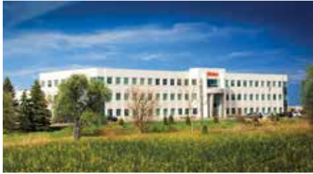
Mitutoyo America Corporation Corporate Headquarters Aurora, Illinois USA
