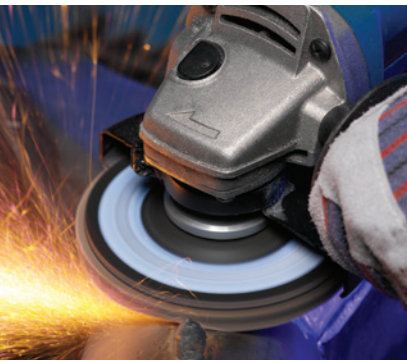
Blending and finishing a weld.
