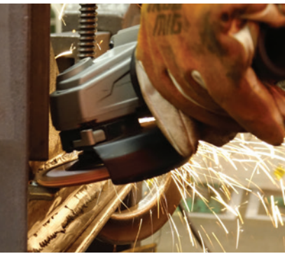
Blending fillet welds to ensure proper penetration prior to inspection.
