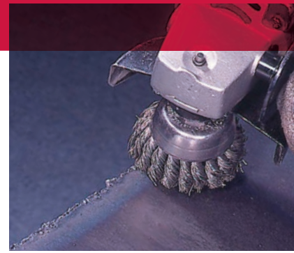
Removing slag from a flame-cut steel plate.
