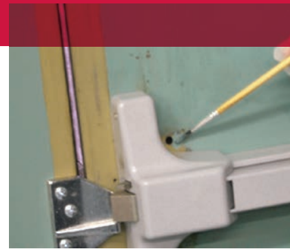
Painting a tight area on a steel door with a Marking Brush.
