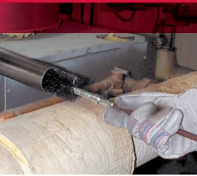
Cleaning boiler pipes with a flue brush.
