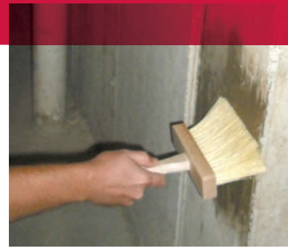
Applying waterproofing material with a masonry brush.
