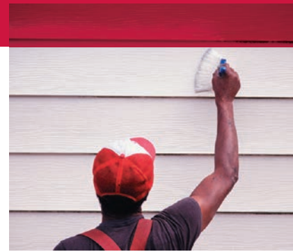
Applying paint to clap board siding.
