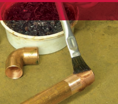
Applying flux to a copper tube prior to soldering.
