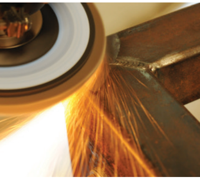
Blending the weld of a steel frame prior to painting.
